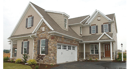
The exterior is stone and Flexlite, with brick accents. There's also a 30-year, textured, dimensional roof; poured-concrete, foundation walls; and a Georgia Pacific floor-joist system that minimizes squeaks.
